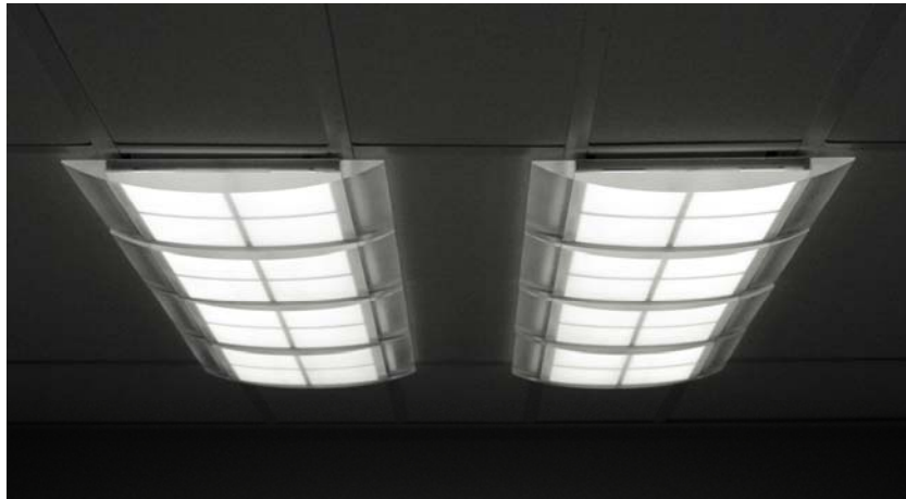
Universal Display PHOLED lighting luminaires mounted in an Armstrong World Industries TechZone Ceiling System. Each luminaire is comprised of four 15cm x 15cm lighting panels mounted in outcoupling enhancement lenses.
